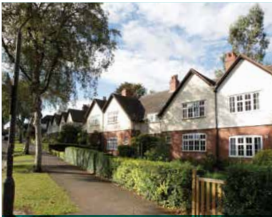
The Moor Pool Garden Suburb in Harborne, Birmingham, is designated a Conservation Area
